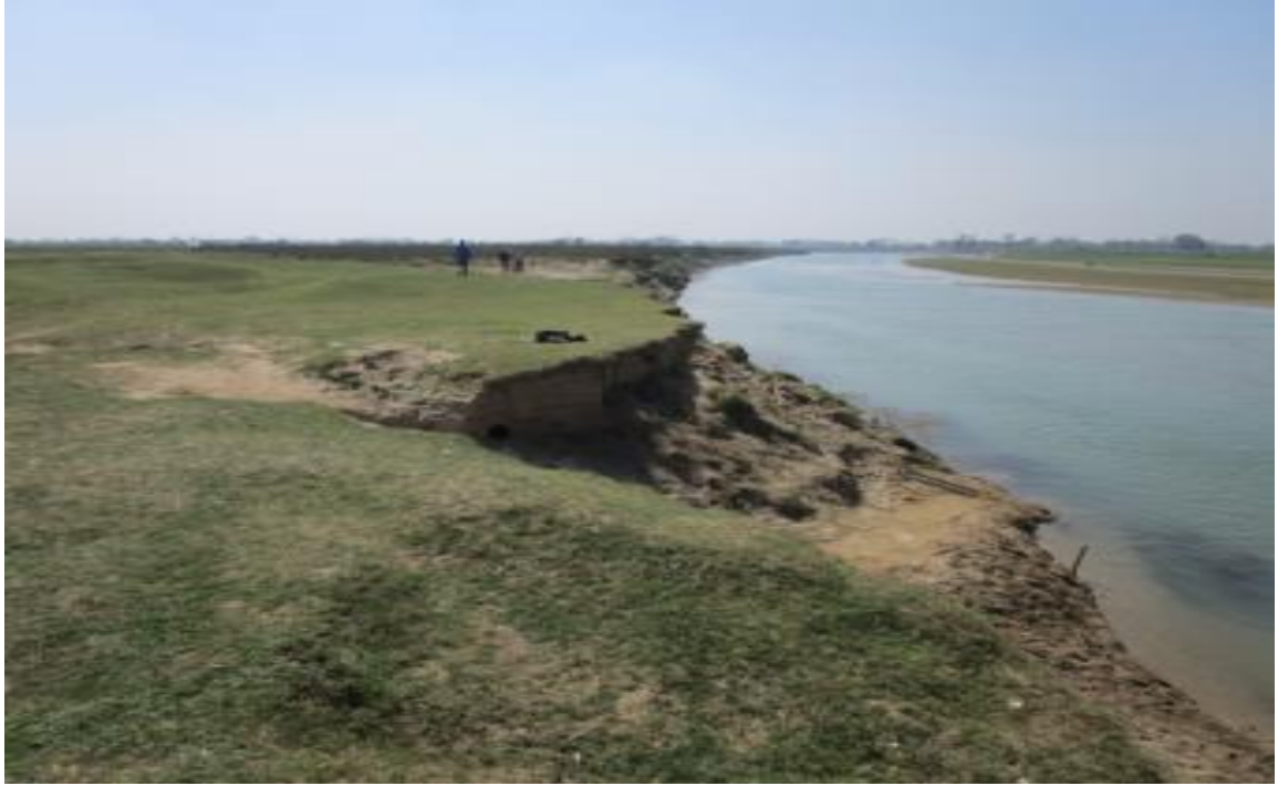
Figure 4: River bank erosion near Kalakunda area (Mohana River)
